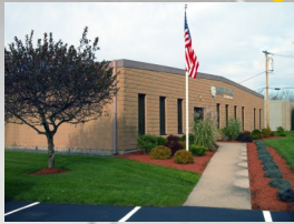
Electro-Fix facility Plainville, MA
